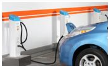
EV Charging Solutions
